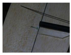
• Trim off the bottom elbow of the control horn, this is required so that the horn doesn't obstruct into the vertical stabilizer when it is pulled forward
